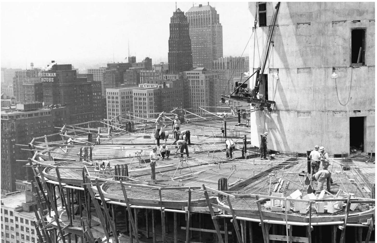
One of Bertrand Goldberg's twin Marina City towers being built in Chicago. When completed in 1968, the towers were the tallest reinforced concrete structures in the world. (Courtesy Geoffrey & Goldberg)
